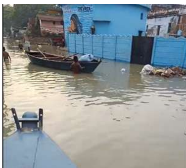
IPS-1 completely submerged in water during peak flood. Backflow issues
