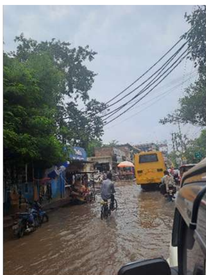
Water logging due to improper planning of drains
