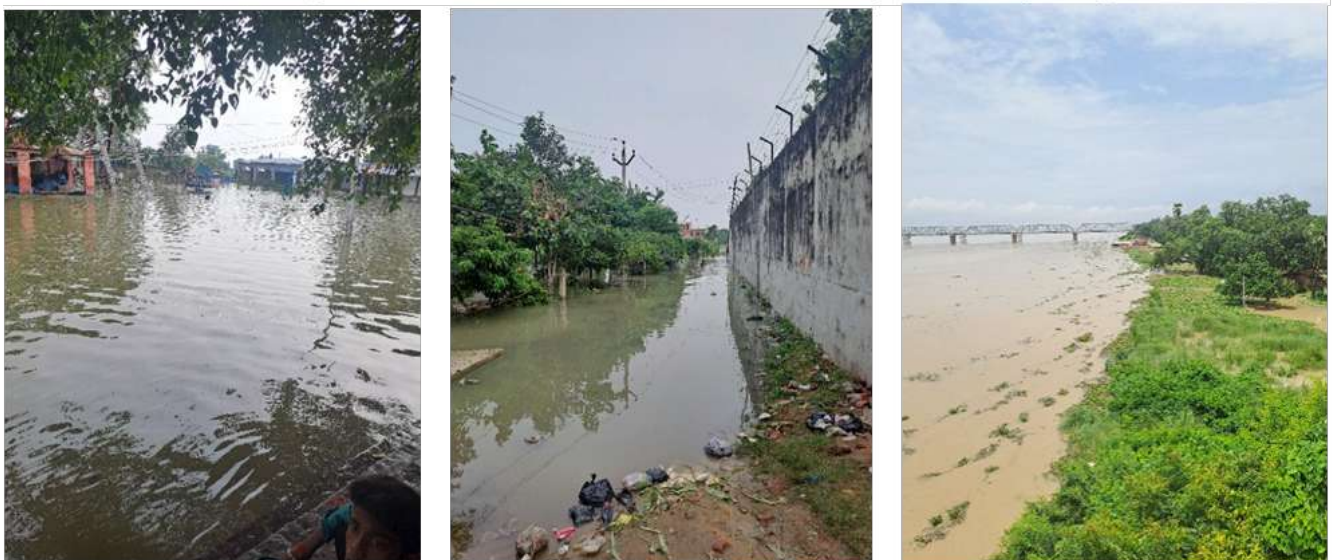
Flooding within the city edge, demonstrating the inundation of the flood. Inundation of Manjhi ghat
